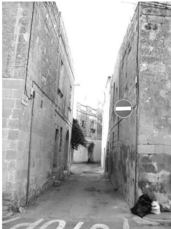
Figure 3: Typical Street that forms part of the Urban Conservation Area in Mosta (MEPA, 2013)
