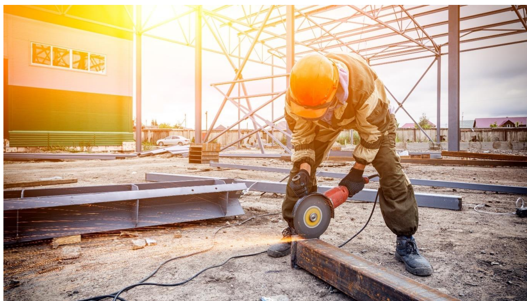
Figure 1 – Cutting steel with a grinder on a construction site (Source: shutterstock.com)
