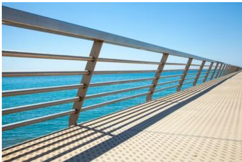
Figure 2 – Metal bridge. (Source: https://shutterstock.com/ )
