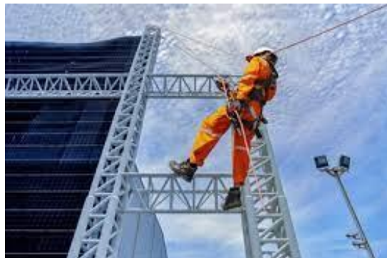
Figure 2: Construction site (Source: shutterstock.com)
