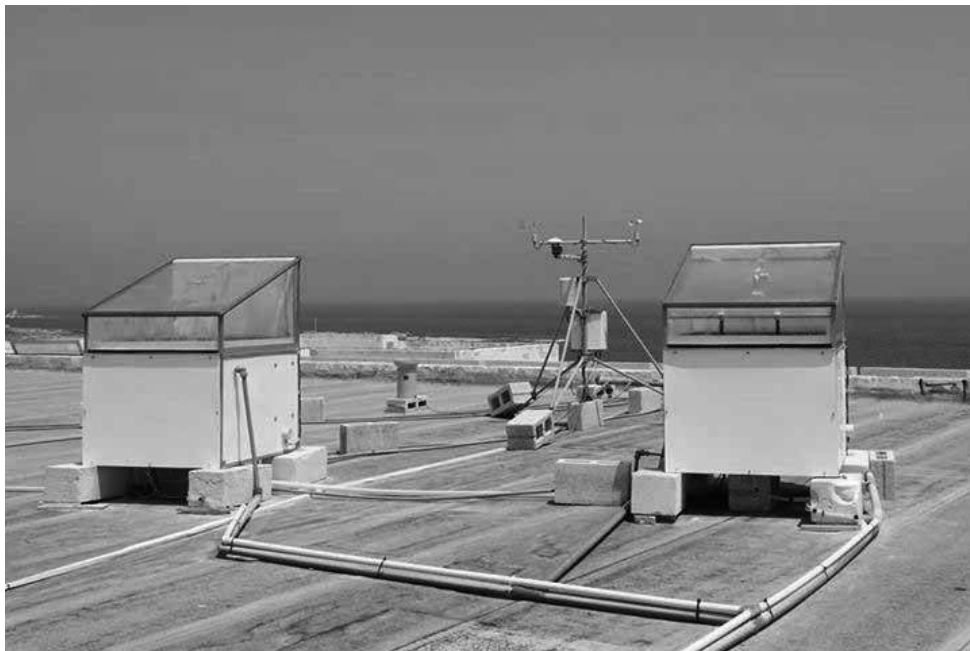
Solar water treatment prototypes tested at Pembroke RO treatment plant
