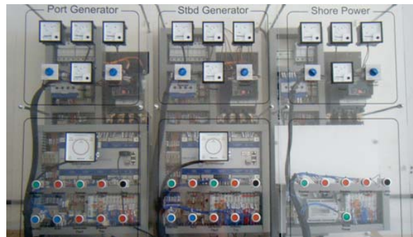
Figure 2: Generator Under Test
