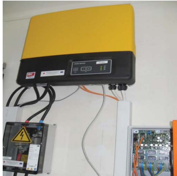
Figure 1: Solar Data Logger: Sunny Boy Control Plus
