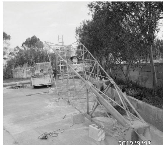
Figure 2: Tower fully assembled on site
