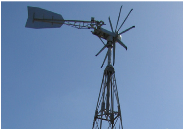
Figure 1: Installed 9-bladed turbine
